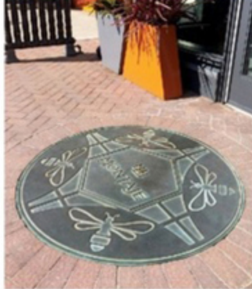
Iron Age collaborated with Seattle-based design firm Foreseer on this custom 4-ft. diameter, cast bronze plaque with antiqued patina finish and highlights for the entry of Montaje, a luxury apartment building in Somerville, Massachusetts.
